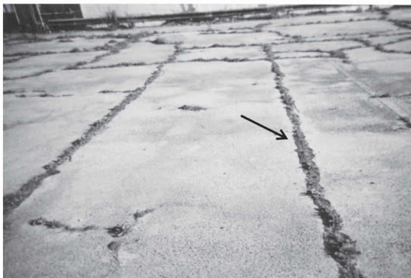
Figure 5. The tar on some of the cracks was used as evidence that these cracks were along seams that had been patched up.
