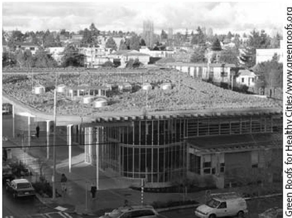
Figure 2: Green Roof on the Seattle Public Library. Photo source: Environmental Protection Agency ( http://www.epa.gov/heatisland/resources/pdf/GreenRoofsCompendium.pdf ), used with permission.
