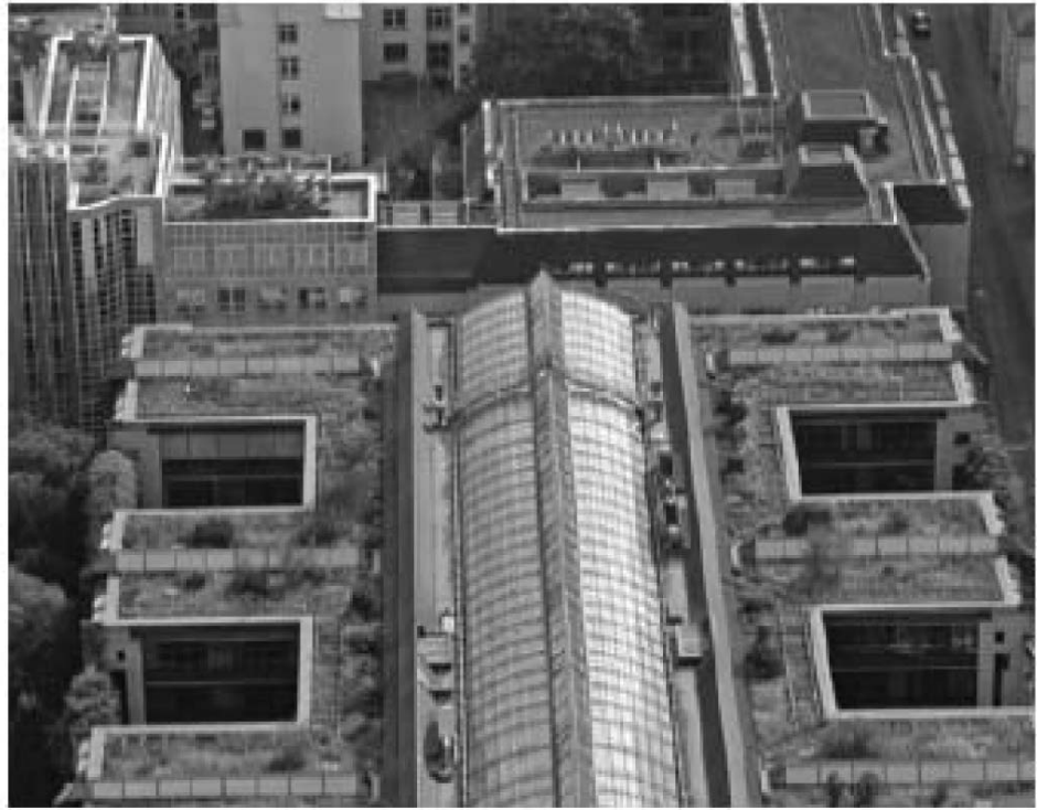
Figure 1: A Green Roof on a Building in Frankfurt, Germany.
